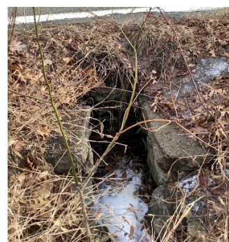
'Failing' Dry Laid Stone
